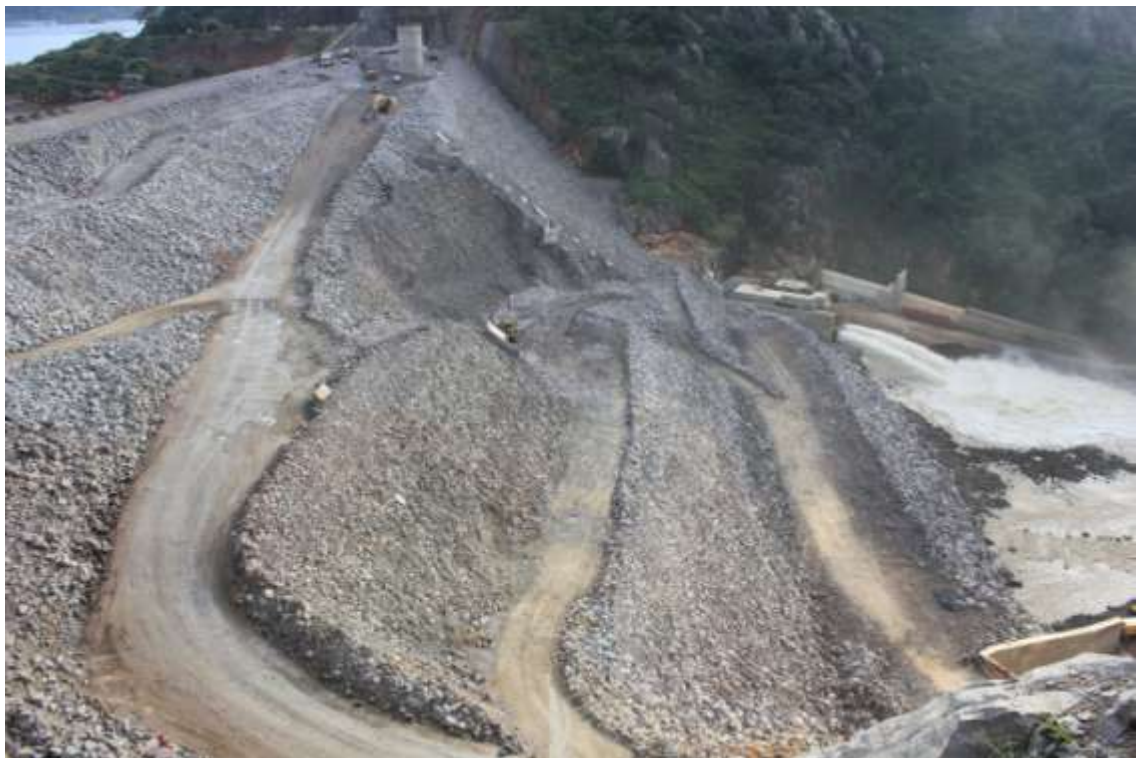
Stabilizing of downstream toe of embankment
