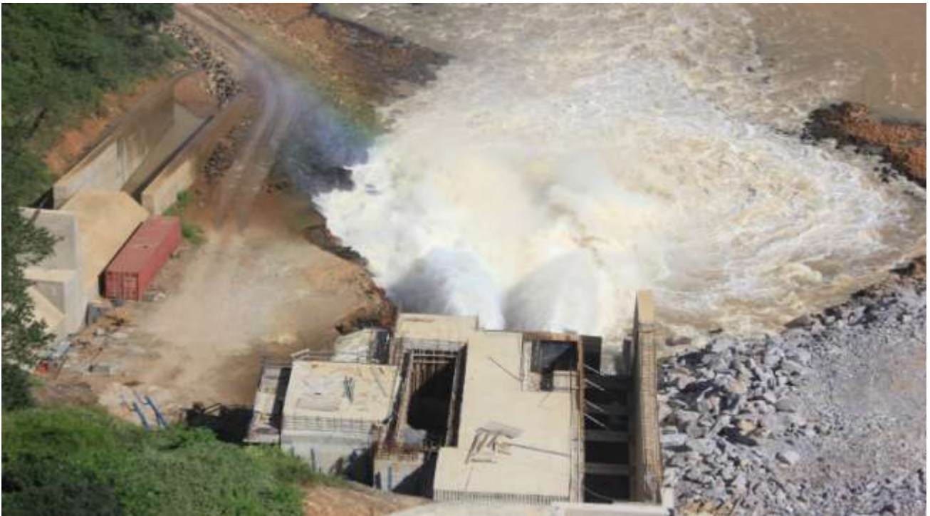
Discharge through the diversion works during and after the floods.
